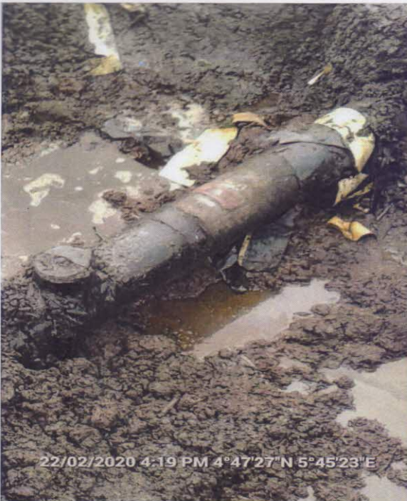
THE POINT AFTER PATCH WELDING.
