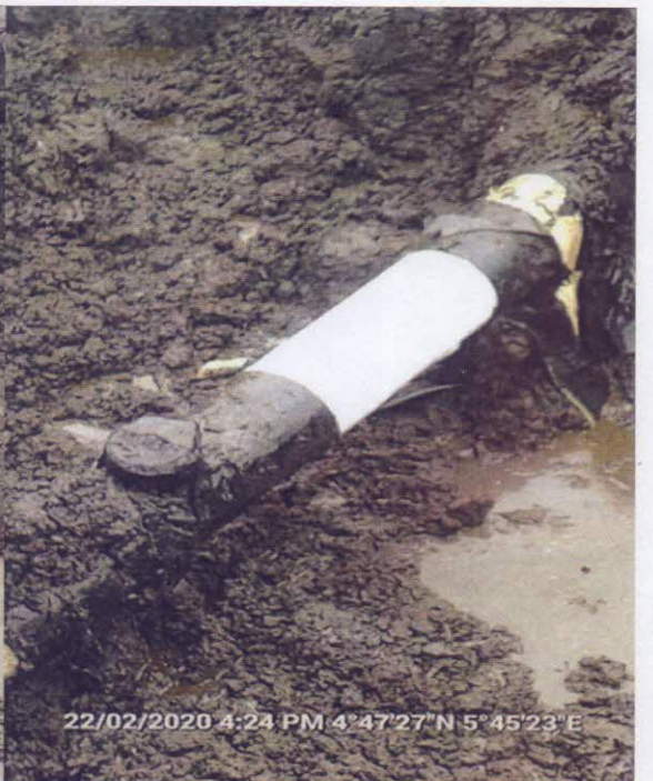
SPILL POINT REPAIRED AND WRAPPED.
