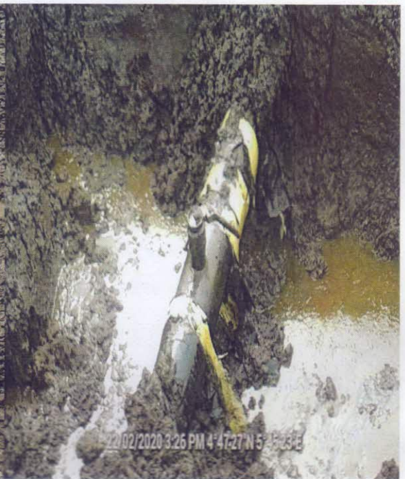
3" VALVE INSTALLED ON THE FACILITY.
